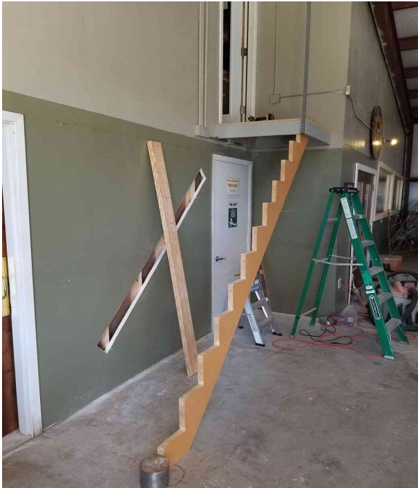
Platform built, suspended, door cut in. Studs located, put in nailer for stringer.
